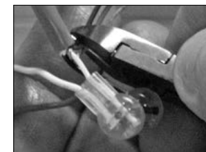
Figure 24- Clip unused wires
