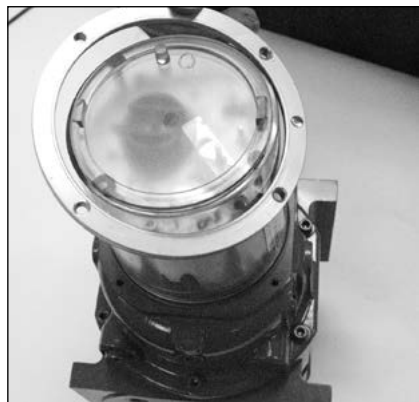
Figure 10.2 - Remove slip flange
